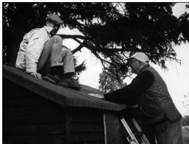
Up on the roof - JB and JW getting felt up.
