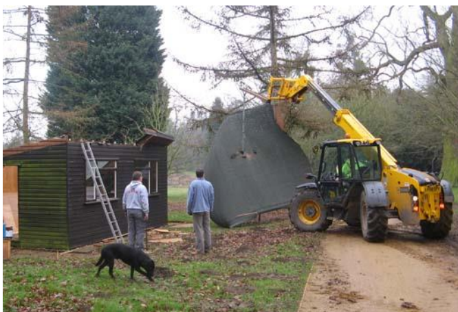
Raising the roof.
