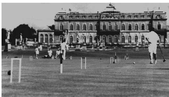
Early morning line-up looking north from lawn 6
